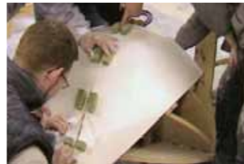
将壳的两部分结合 Applying DuPont™ Corian® joint adhesive to the seam
